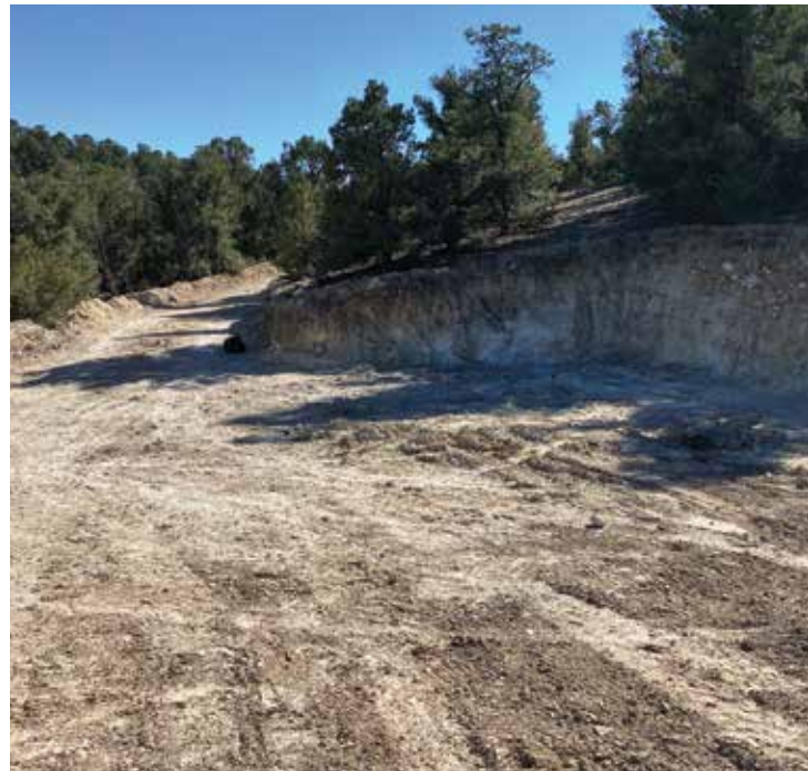
Drill pad with road leading to it. Lynn Boulton
