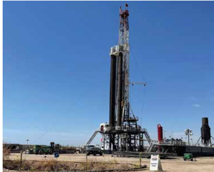
Drilling for lithium brine in Imperial Valley.
